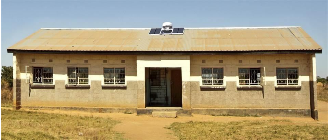
Figure 1.1 Rural School User Terminal Example with Solar Power
